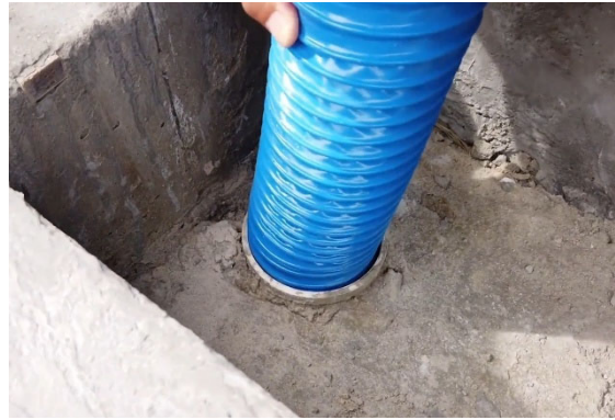
Connect the drain pipe
