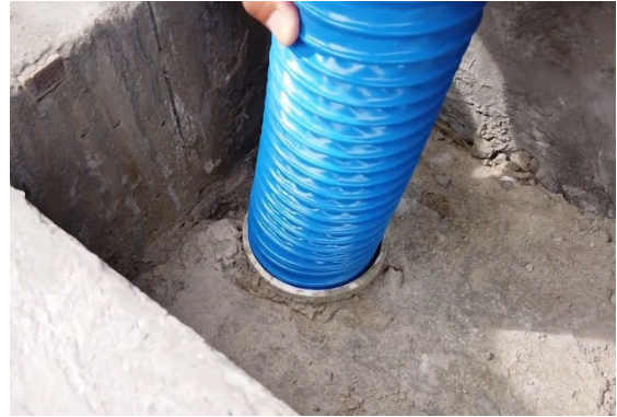
Connect the drain pipe
